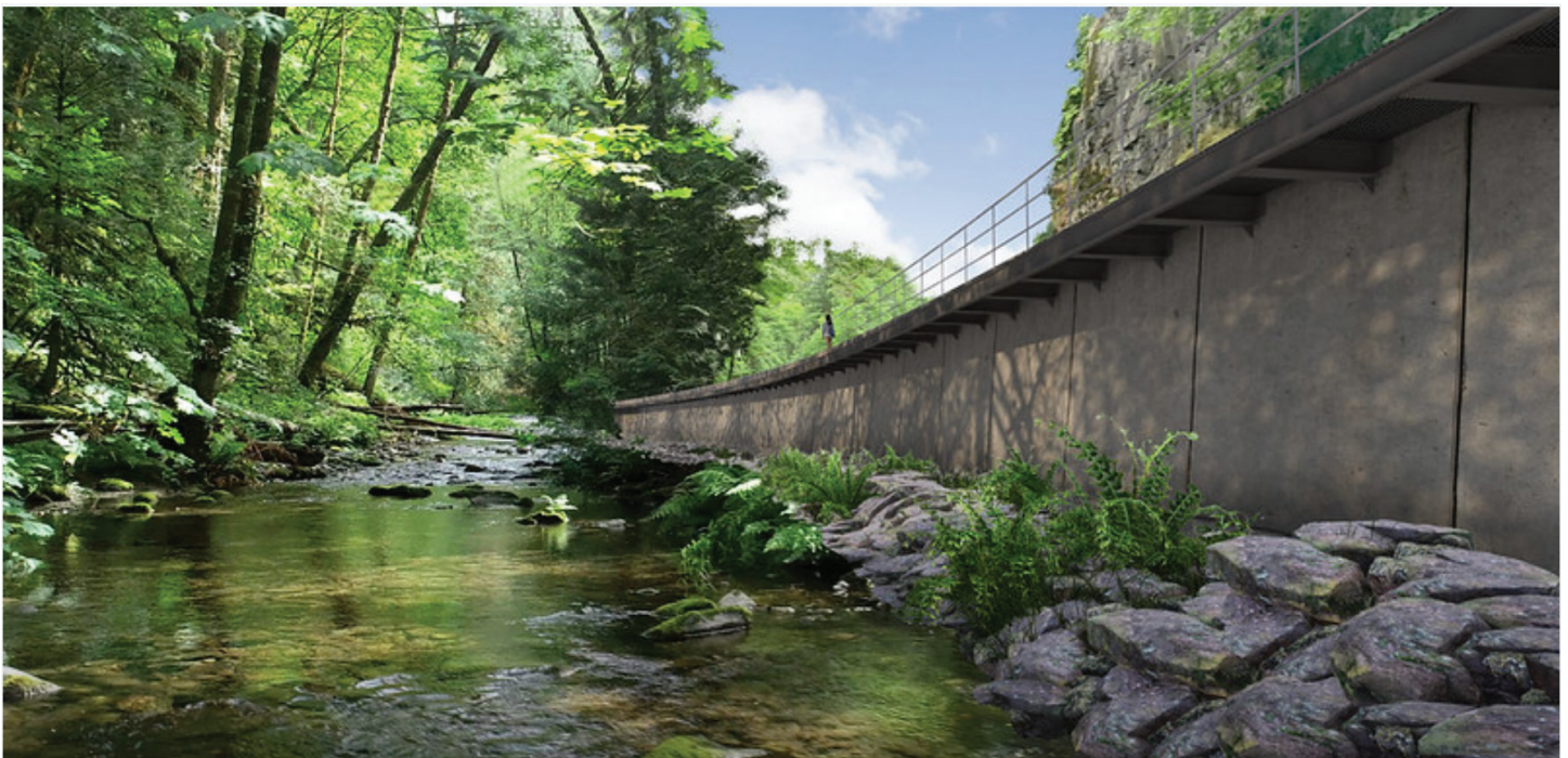
Rendering of Highway 1 retaining wall within the riverbank and habitat restoration once complete (looking south). Retaining structures are proposed at two locations along the river within the 2.2 km Project length – one would be 54 metres long and one would be 144-metres long.
